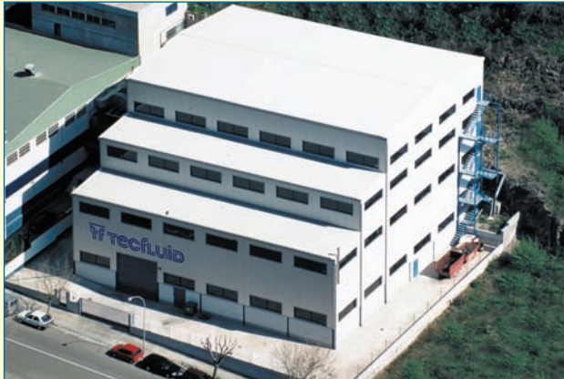
R+D, Manufacturing and assembly workshop
